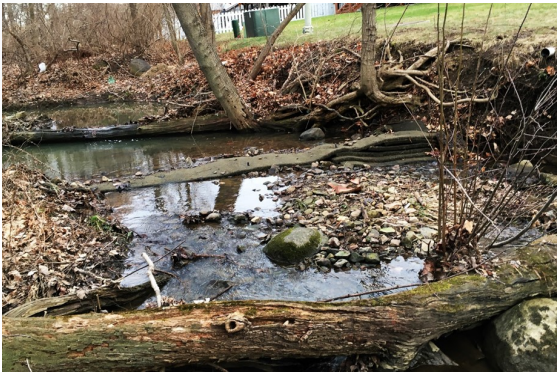
A stream insert oriented to move water away from the eroding bank on the right.
