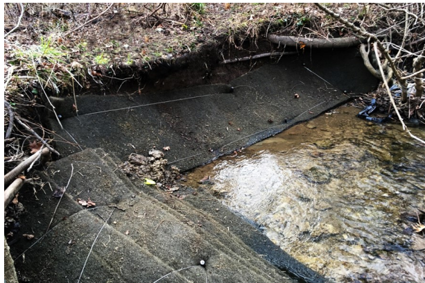
Insert material placed to reduce erosion at a bend.
