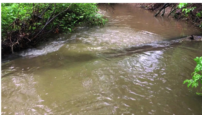
Water flowing over insert oriented to reduce erosion on right bank.
