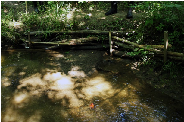
Wood placed to reduce bank erosion at a bend.
